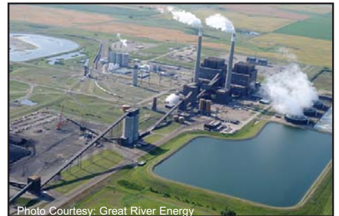
Coal Creek Station
