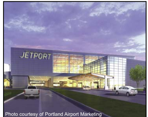
Airport Terminal Expansion Portland, Maine
