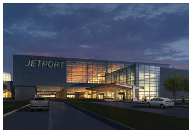
Airport Terminal Expansion - Portland, ME
