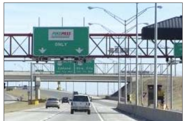
Oklahoma Transportation Authority Turnpike System
