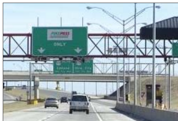
Oklahoma Transportation Authority Turnpike System
